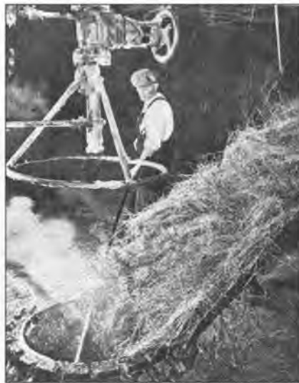
Esparto grass being fed to the boilers
